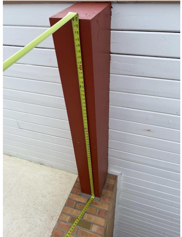
Item S4 – Typical roof framing cantilever outside Main Level Classroom space.
