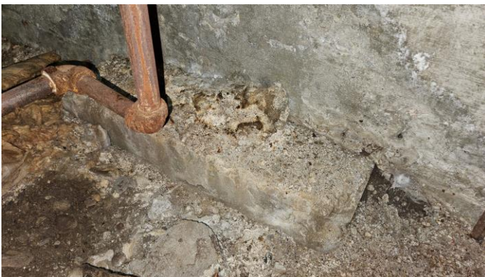
Item S1 – Typical spread footing below masonry pilaster at Main Level Classrooms.
