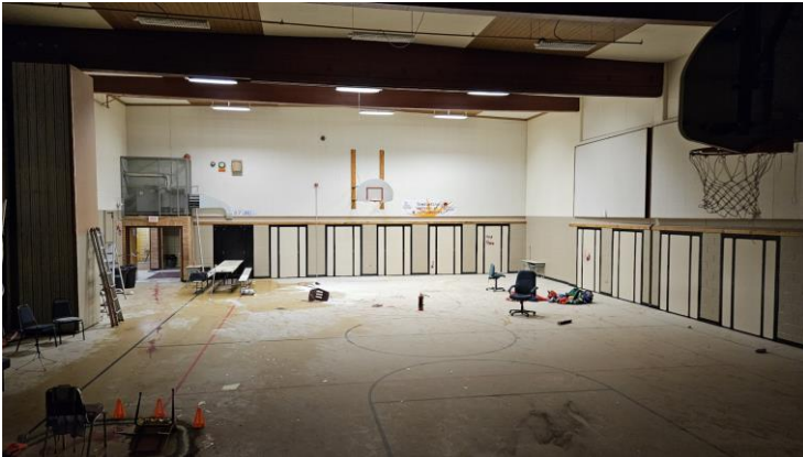
Item S7 – View of gymnasium, looking North from stage.
