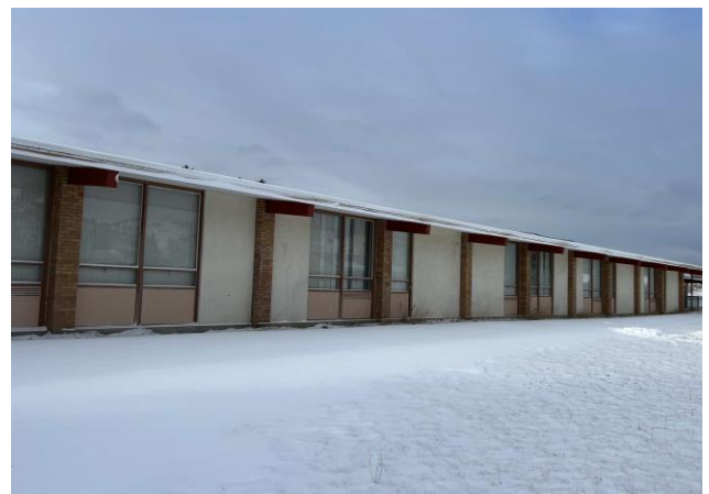
Item S3 – North exterior wall line of Main Level Classroom space. Full height walls present between window openings.
