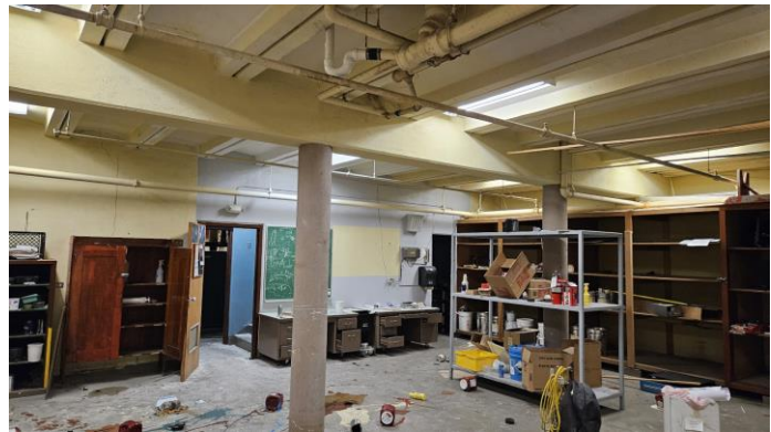
Item S6 – Typical floor construction above Room 011. Precast Longspan Channel Slab planks spanning to interior beam / column line.
