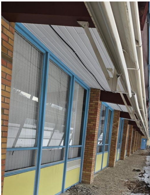
Item S3 – South exterior wall line of Main Level Classroom space. Limited full height wall present on this line.
