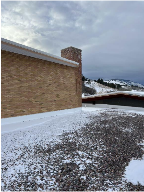
Item S8 – Ballasted lower roof, North of upper gym roof.
