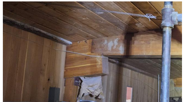
Item S4 – Classroom roof beam support and hallway beam connection at edge of Hall 113.
