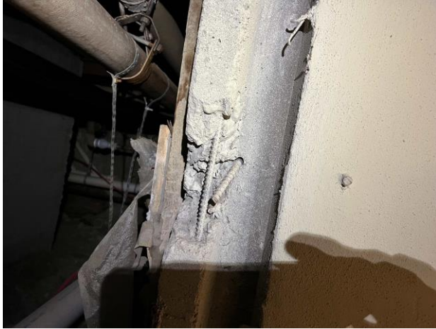
Item S1 – Typical Main Level Classroom Foundation wall. Reinforcing steel protruding from wall.
