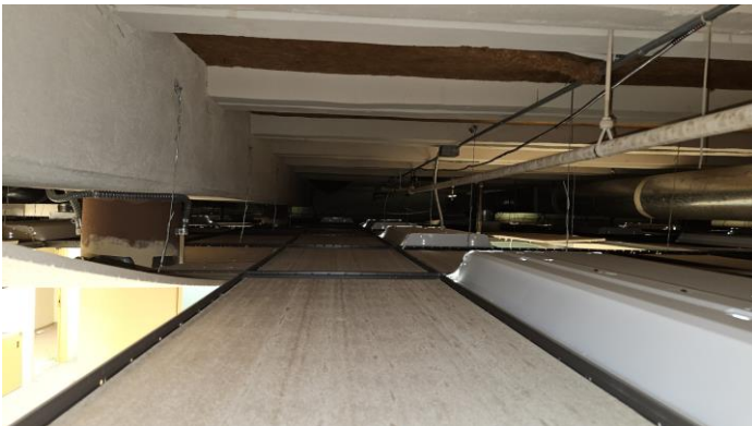
Item S6 – Typical gym floor construction above Room 003 at interior beam / column bearing line.
