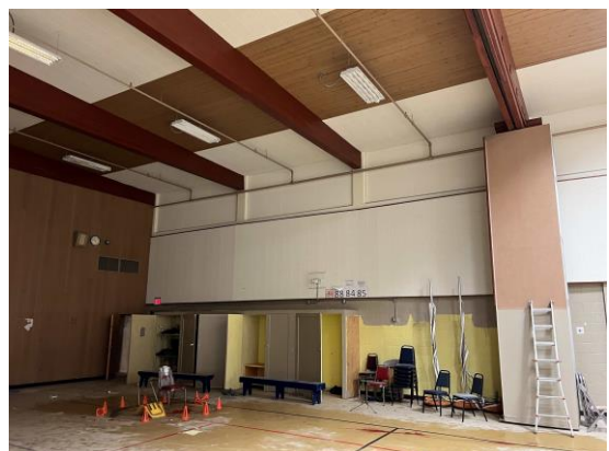
Item S8 – Typical gym roof framing. Car decking spanning between tapered glulam girders that reside on CMU pilasters.
