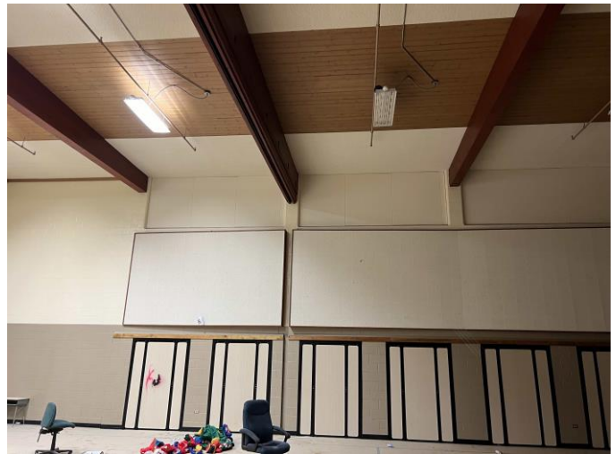
Item S7 – North half of East gym wall. Full height CMU wall section can be seen to left with partial-height infill shown (3) bays to the right.
