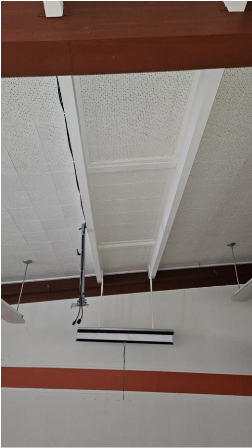
Item S4 – Typical roof framing observed from within classroom space.
